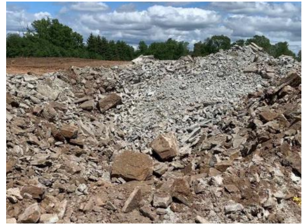
Aftermath of rock blasting (6/21/2021)
