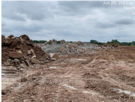
Piles of rock from the blasting activities (6/28/2021)
