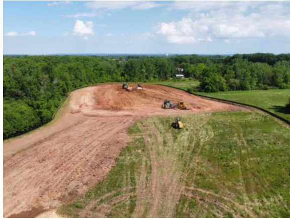
Retention ponds start to get shaped (6/1/2021)
