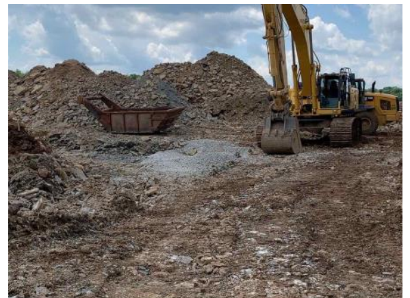
Deep sanitary excavation starting at manhole 19 (6/30/2021)
