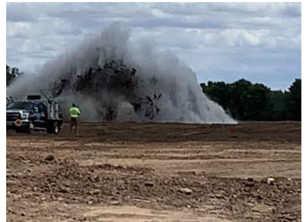
Still photo of rock blasting (6/23/2021)
