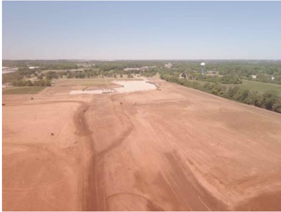
Aerial photo of the North half of the site (6/16/2021)
