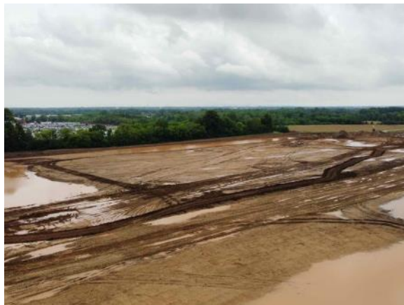
Wet conditions after a rain day (6/29/2021)
