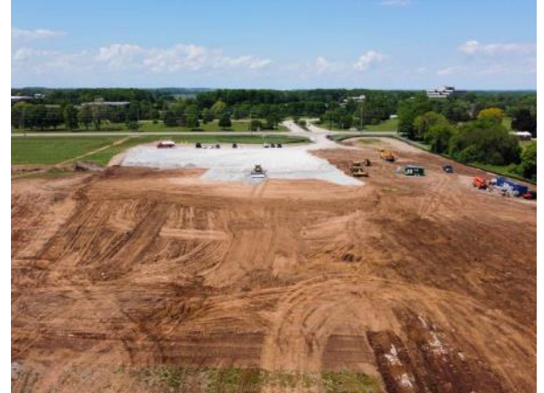
Parking lot stone is leveled and earthwork starts (6/1/2021)
