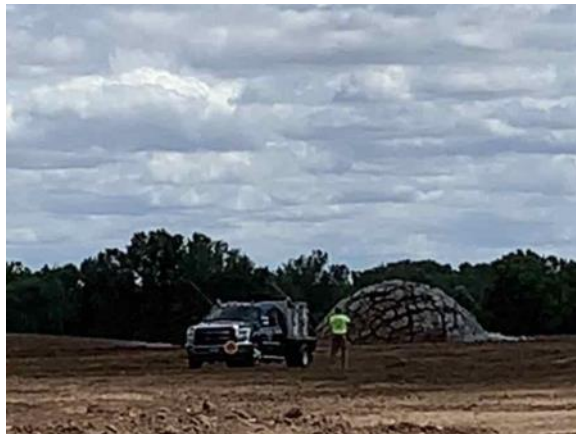
Still photo of rock blasting (6/23/2021)
