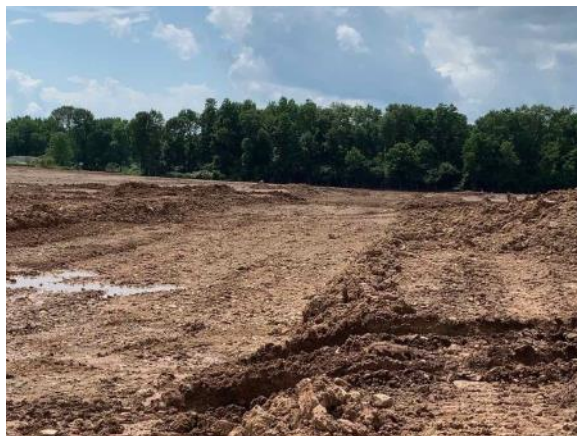
Future road between the soccer and baseball fields (6/30/2021)
