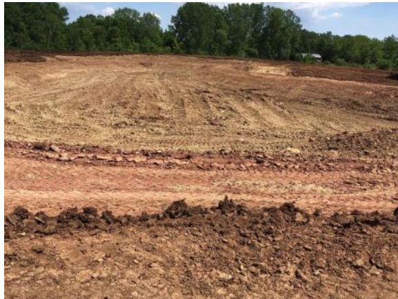
Retention ponds taking shape (6/2/2021)
