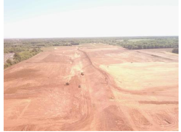
Aerial photo looking South (6/16/2021)
